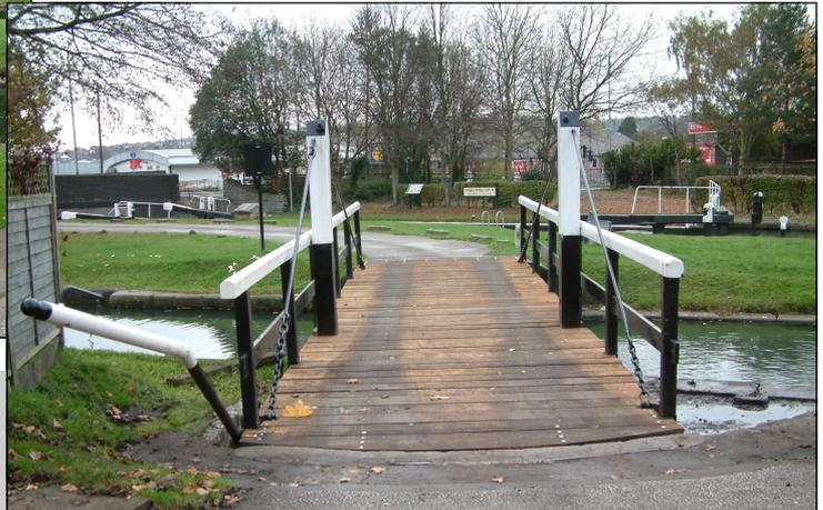
**Erewash Canal Preservation Development Association** have recently been involved in refurbishment of the Langley Mill swing bridge under a contract with British Waterways (East Midlands). It was originally made in 1986, replacing a wooden structure. A lot of welding and new steel was needed as much of it especially in the weight section had deteriorated due to water ingress.
