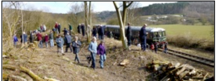
The CVR train with passengers exploring the site of Johnsons Lock on the Uttoxeter Canal restoration.
